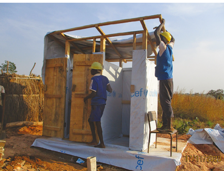
Building semi-permanent latrines, Canaa District, Bambari. CAR – © TGH
