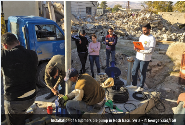
Installation of a submersible pump in Hosh Nasri, Syria - © George Saad/TGH
