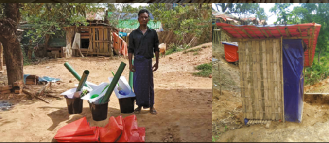
Distribution and installation of emergency latrine kits in Samee, Myanmar – © RCDF/TGH
